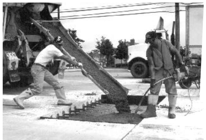
Figure 8: Placing concrete during full-depth repair.
