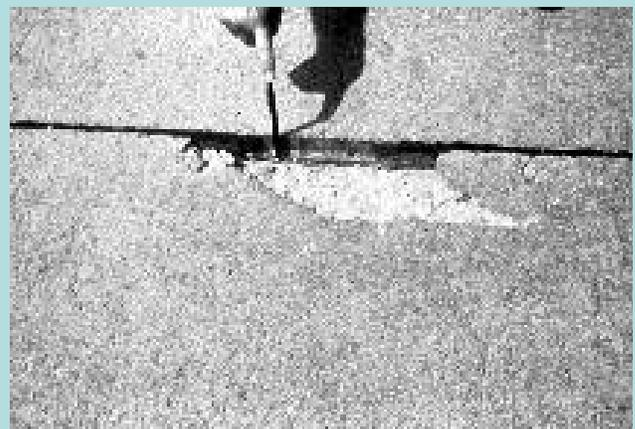
Figure 4: Slab with moderate deterioration.
