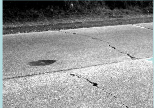
Figure 2: Cracked slabs with low deterioration.
