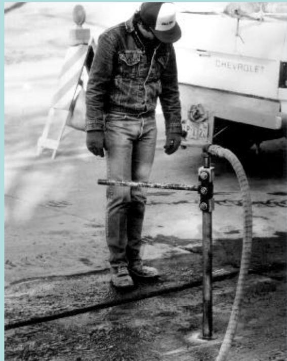
Figure 11: Slab stabilization.
