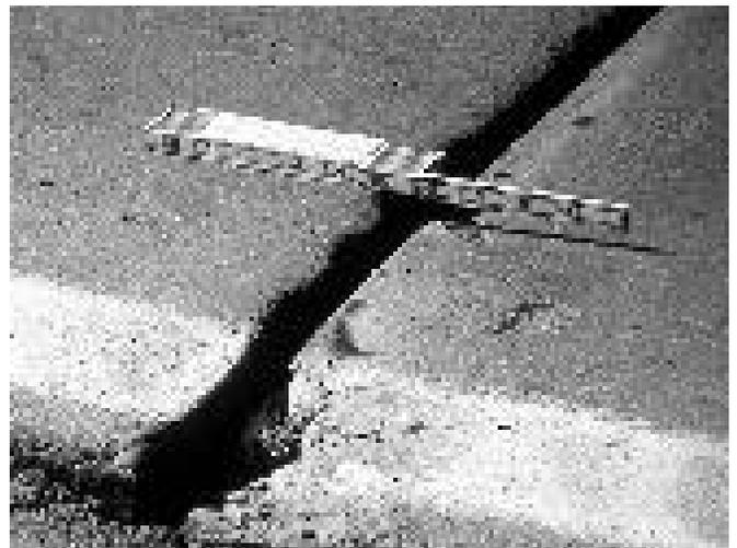
Figure 6: Faulted joint.
